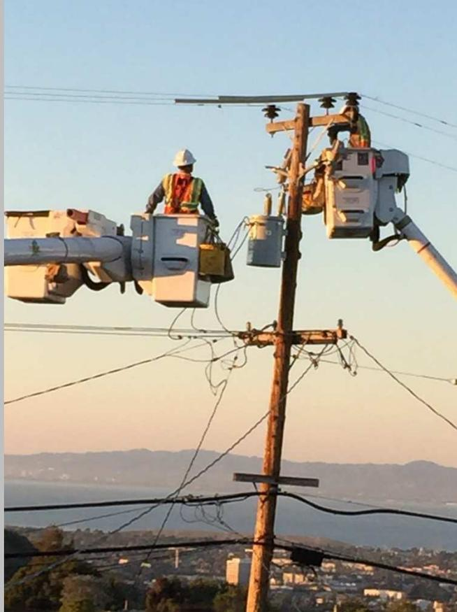
**51 year old transformer was leaking – replaced with new transformer**
